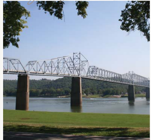
Milton Madison Bridge over the Ohio River between Kentucky and Indiana (photo courtesy Wilbur Smith Associates/Michael Baker Engineers)
